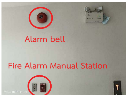
Alarm bell & Fire Alarm Manual Station
